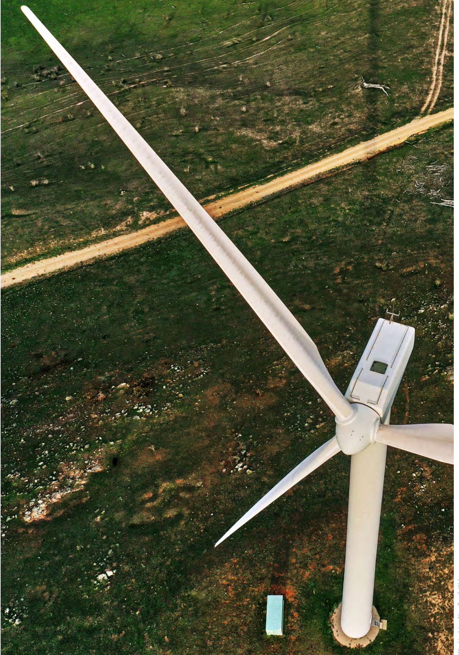
Wind turbine, New South Wales.
